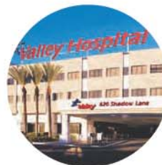
Valley Hospital Medical Center
